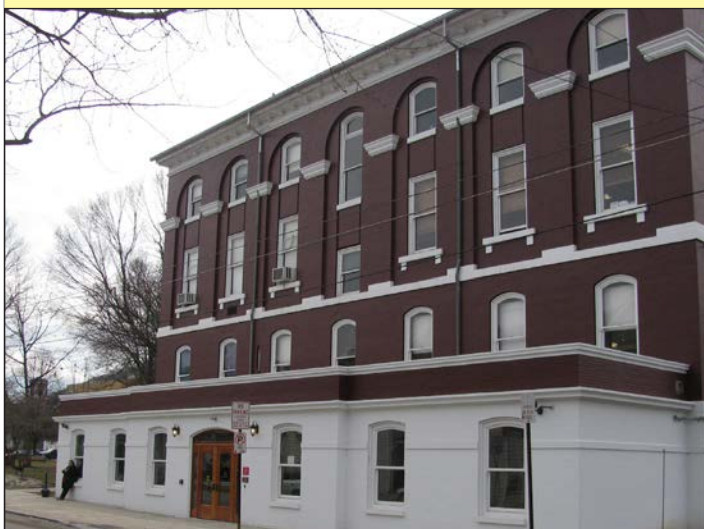
$16,141 was spent at the Venango County Courthouse for architectural barrier removal.
