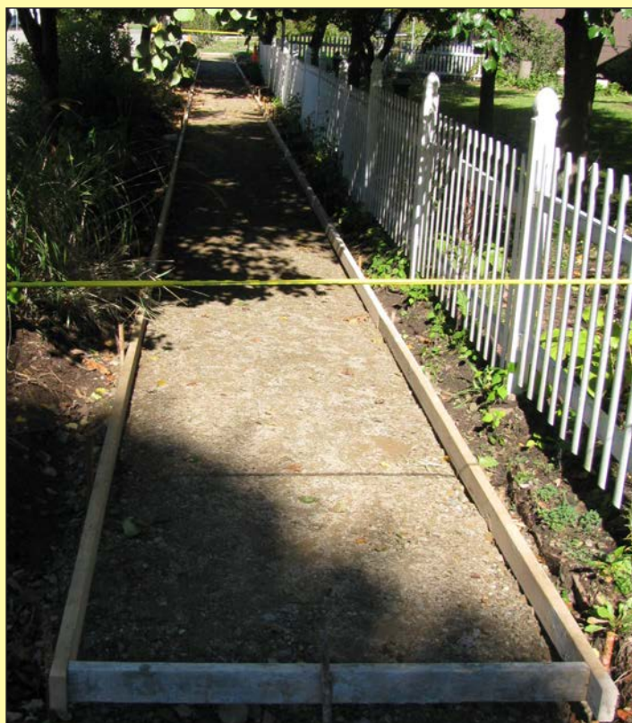
$380,000 was spent in Utica Borough for the construction of new sidewalks.
